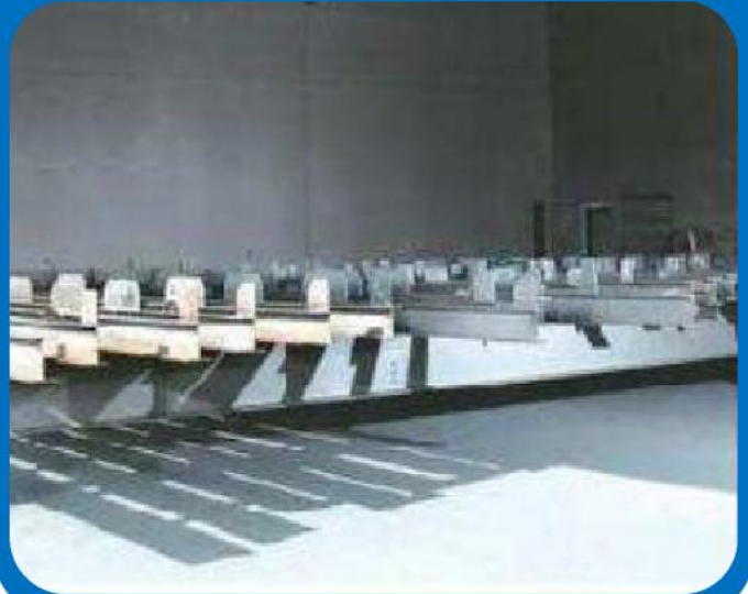
SHOT BLAST ROOM
