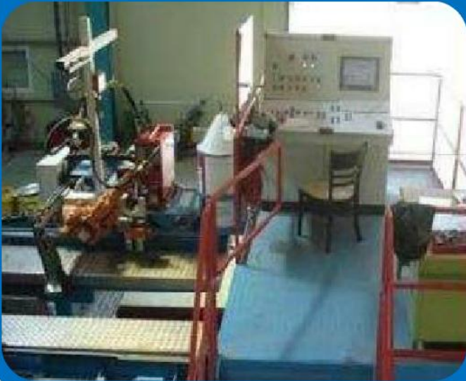
Main control booth
