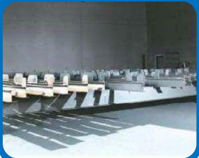
SHOT BLAST ROOM
